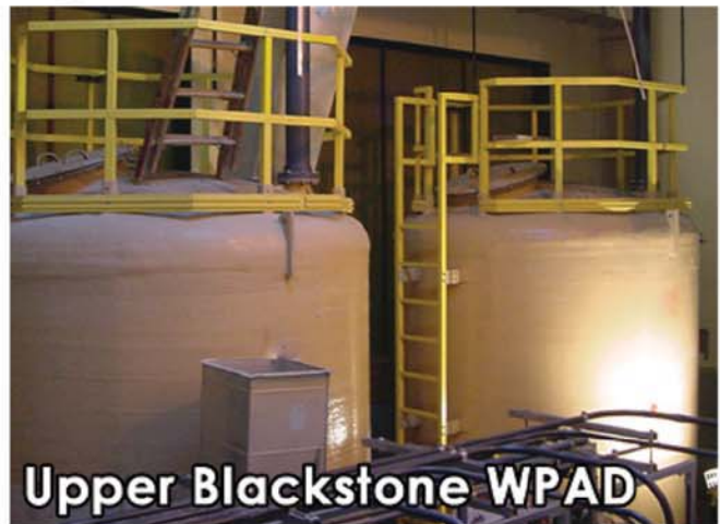
FRP chemical feed tanks were supplied to the Upper Blackstone Water Pollution Abatement District with FRPI Certification. District Engineer Karla Sangrey was so satisfied with the results that she joined the FRPI Board of Advisors.
